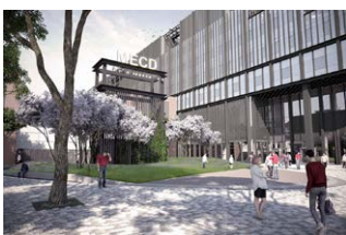
Manchester Engineering Campus Development, UK
